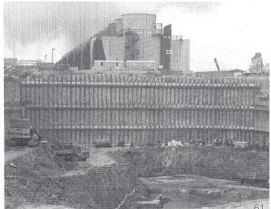
Anchored bored pile Wall Neckarwestheim nuclear power plant 1983
